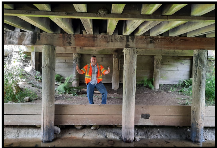
Thomas Creek Bridge – Old Hwy 99 N.
