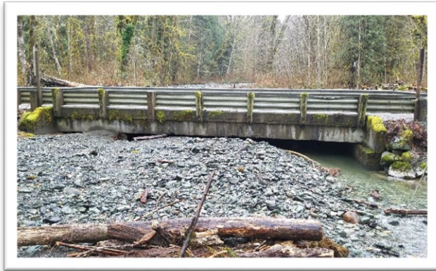
Mill Creek Bridge – South Skagit Highway
