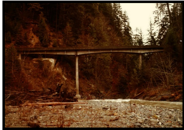
Upper Finney Creek Bridge – Finney Creek
