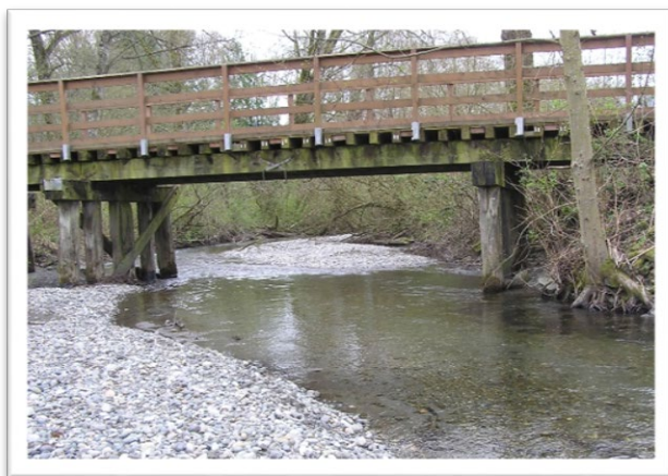
Cascade Trail Bridge over Jones Creek
