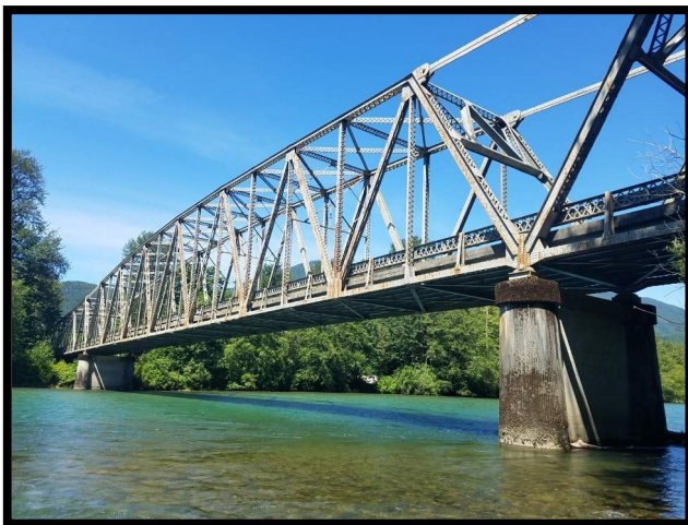
Marblemount Bridge – Skagit River
