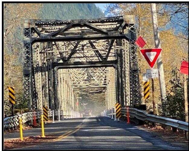
Marblemount Bridge – Skagit River
