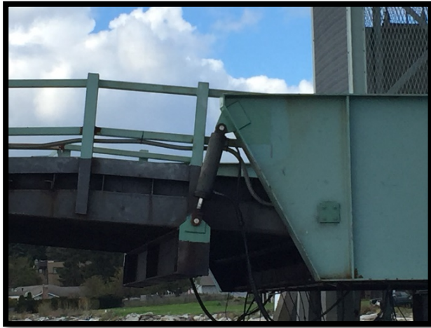
Guemes Island Terminal – Transfer Span
