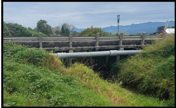
Thomas Creek Bridge – Old Hwy 99 N.
