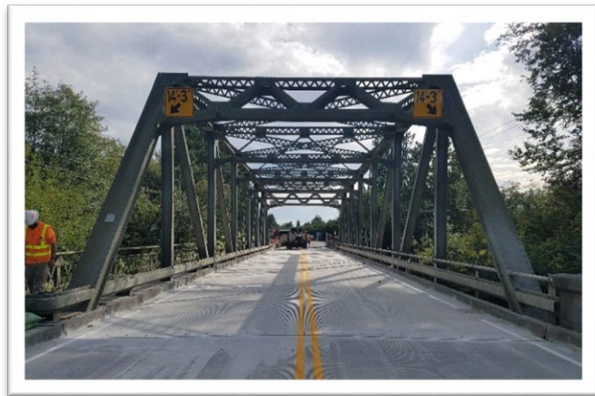
Samish River Bridge - Vertical Clearance Signage
